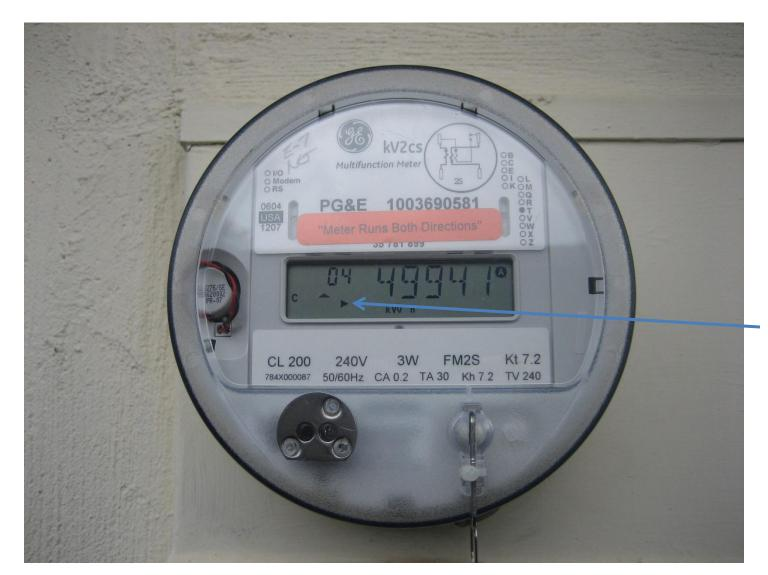
•Meter initially set to 50,000 kWh •On 3/30/10, produced 59 kWh more power than consumed •Arrow pointing to the right indicates that power is flowing into the home
